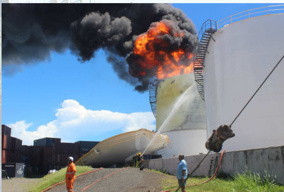
Samoa, 4 april 2016, dieseltank (Ø 15 meter)
