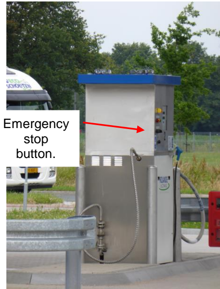
Supply point with emergency stop button.
