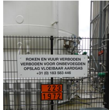
Recognisability of LNG & contact details of operator in the vicinity of the storage tank.
