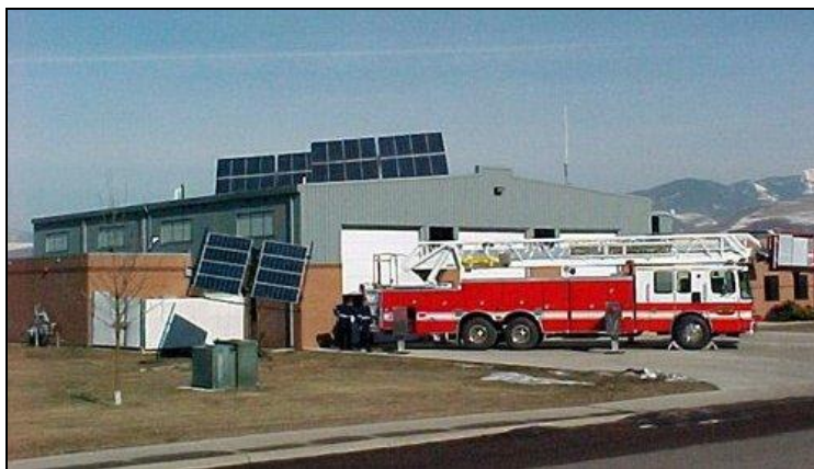
Figure 2-7: Example of Fire Station with a Photovoltaic Solar Power System in Missoula, MT (Photo courtesy of NREL Photographic Information Exchange)
