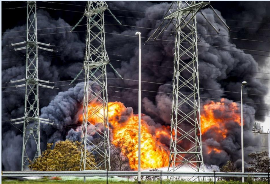
Brand op Chemelot terrein, 9 november 2015 [35]
